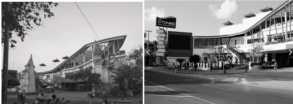
Gambar 4. Dinding Fasad Hotel The Stones Sumber: Data Pribadi (2019)
